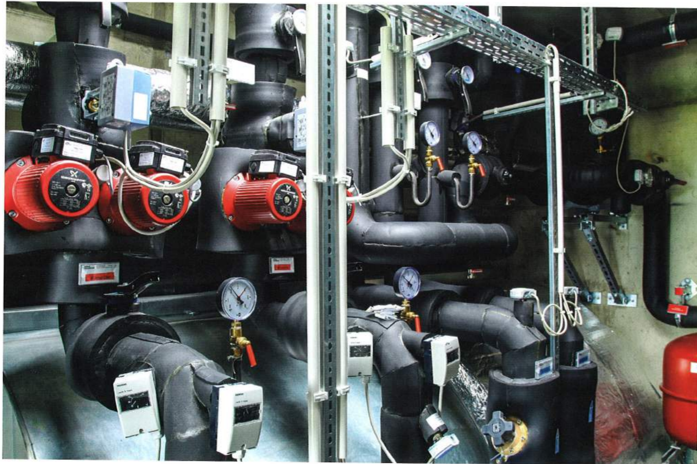
Desigo controls the concrete core tempering system via the Desigo TABS Control application.
